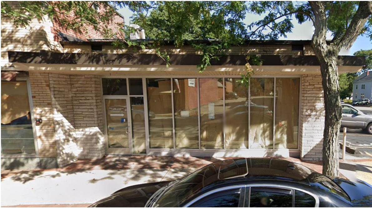
Previous/Existing front view
